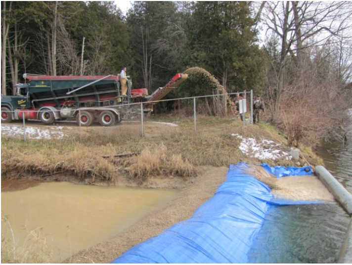
A new trash boom was put in place and a temporary berm was constructed to hold back the water. The top and bottom plates were then removed.
