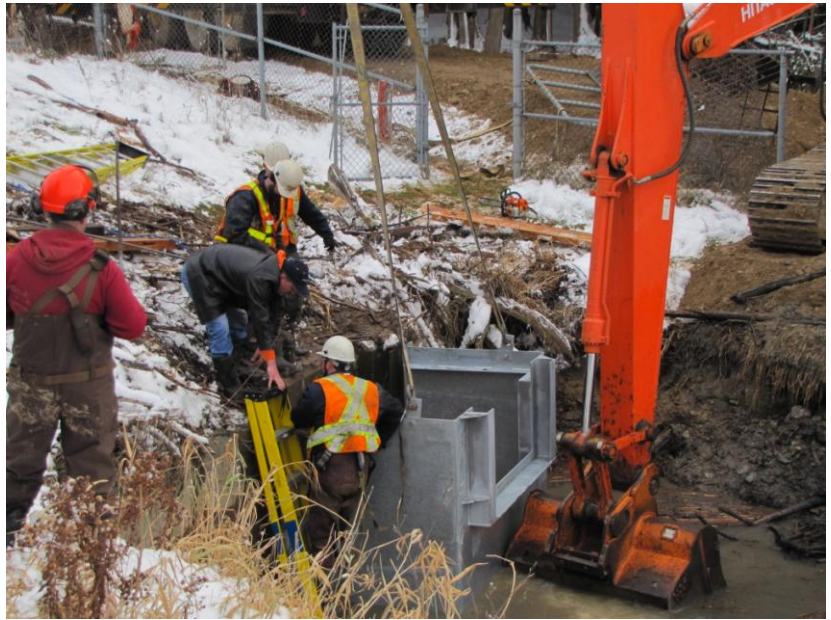
The engineered flow-control device which can be adjusted for optimum flow rates is carefully hoisted in place and anchored.
