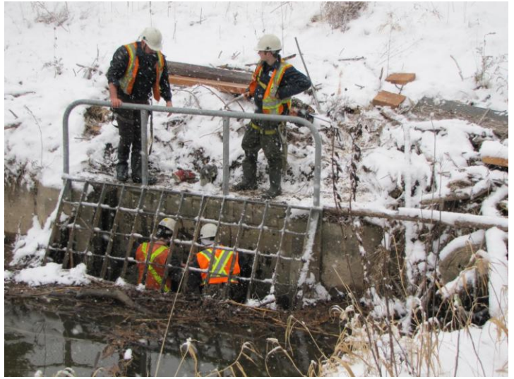
A new trash boom was put in place and a temporary berm was constructed to hold back the water. The top and bottom plates were then removed.
