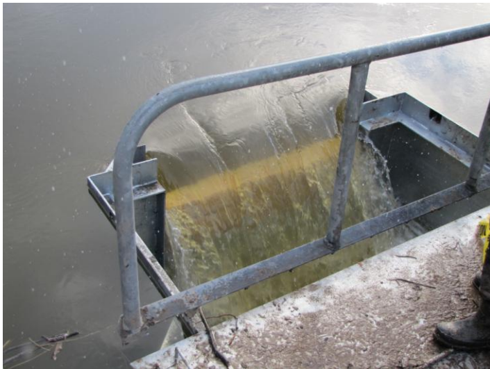
The berm is removed and optimum flow is restored to the upper entrance (left) creating a much improved, and now easily-negotiated lower entrance.
