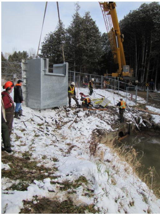
The engineered flow-control device which can be adjusted for optimum flow rates is carefully hoisted in place and anchored.
