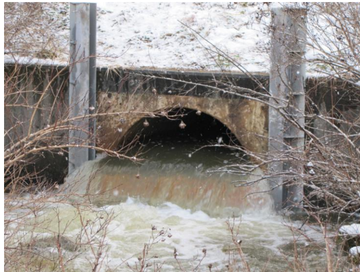
The berm is removed and optimum flow is restored to the upper entrance (left) creating a much improved, and now easily-negotiated lower entrance.
